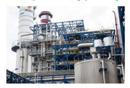
The EUR 75,000 project aimed at installing an efficient and effective technical solution to reduce steam consumption at the gas turbine firing system in the cogeneration unit. Consequently, an annual steam reduction of around 22,000 GJ was achieved, equivalent to a  $\rm CO_2$  reduction of around 1,200 t per year.
