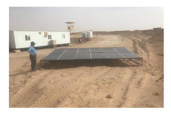
OMV Security teams in Yemen initiated the installation of solar power at the permanent checkpoints and guard positions around its concession in Shabwa, Yemen. Solar power will be used to power the facilities and provide lighting, electricity, and heating while reducing carbon emissions, maintenance, and fuel costs incurred in running fossil-fuel generators.
